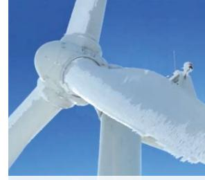
Ice accumulation on the rotorblade
